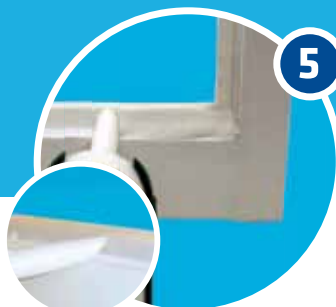
Cut the nozzle to form the glazing profile and apply DRY SEAL™
